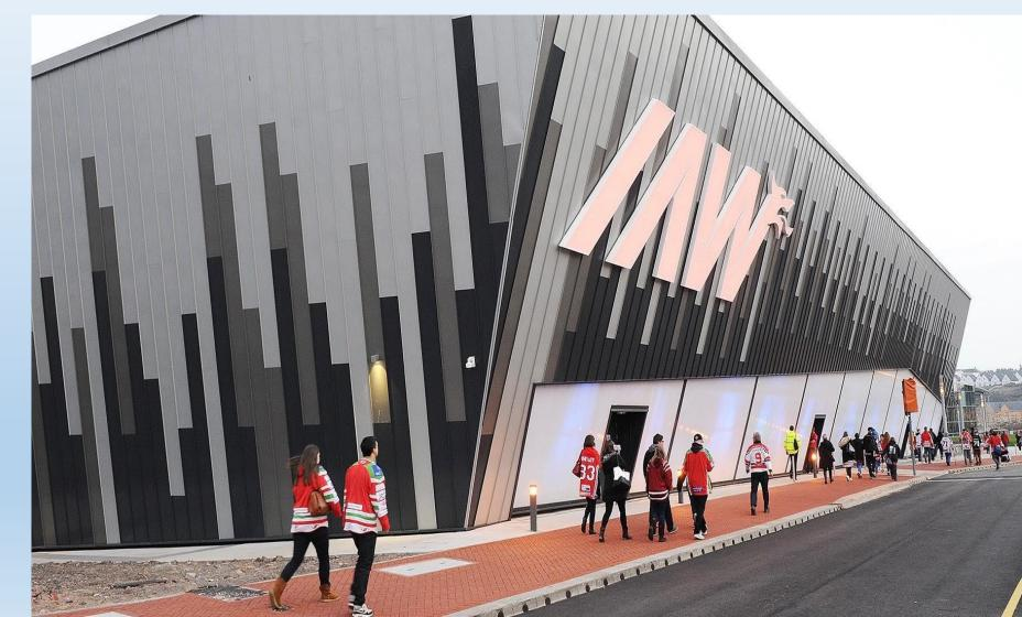
It is a striking building of steel frame construction with dark to silver metal cladding with a gently raked roofs with angled walls that give the building a distinct character which extends to approximately 8,336m<sup>2</sup> (89,728 ft<sup>2</sup>) Gross Internal Area (including areas of plant and services).
